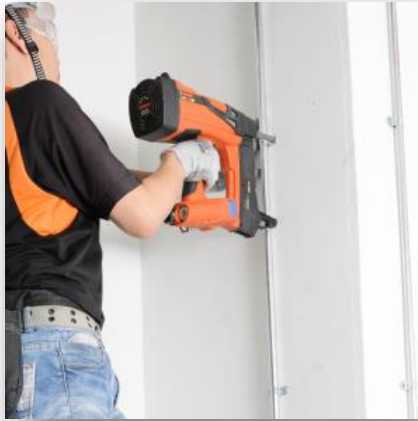
Fixing electrical conduit clips & trunking systems
