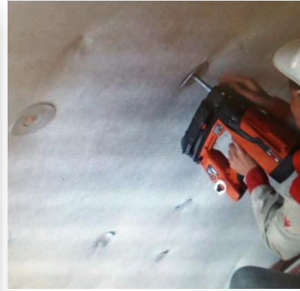
Fixing water-proofing membrane to tunnels
