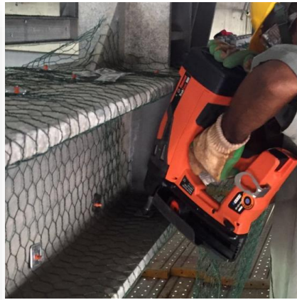
Fixing wire mesh to structural steel
