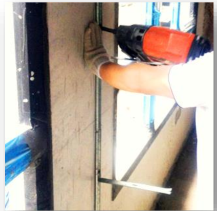
Fixing wall-tie & bonding bar system
