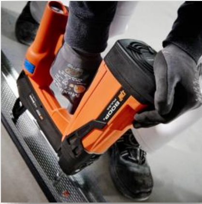
Fixing drywall tracks to concrete & steel
