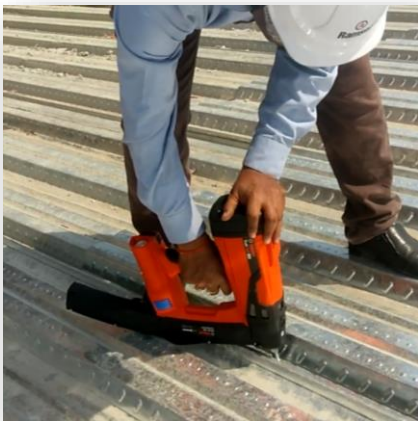
Fixing structural steel decking sheets on structural steel
